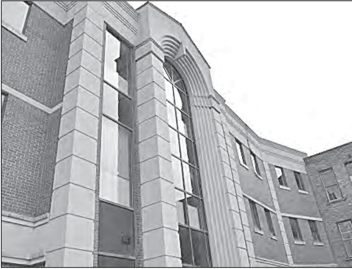
The building that once housed SUNY Morrisville's remote campus is likely to be repurposed as a boutique hotel in downtown Norwich. The project is one of nine in the city identified by Commerce Chenango that will greatly benefit from the $10 million Downtown Revitalization Grant awarded by New York State. (Photo by Shawn Magrath)
