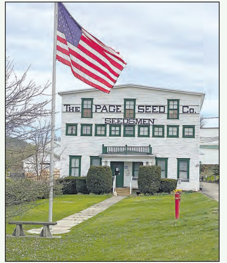
The Page Seed Company, located in Greene, NY, has expanded their production space by utilizing a previous storage area. The construction is a five year project and will offer new jobs with more machinery and equipment which will increase employment opportunities. (Photo by Kelli Miller)
